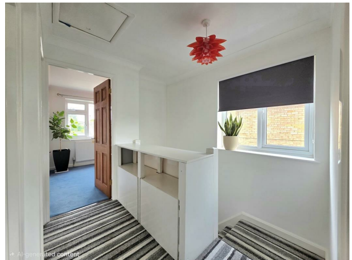
Upvc window to side elevation. Loft Access. Skimmed ceiling. Built in storage.
