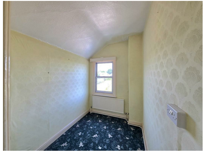
PVC double glazed window to rear. Radiator.
