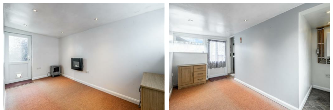
UPVC Double glazed window and door to front and rear. Electric fire. Space for tumble dryer. Space for fridge/freezer. Mains gas central heating boiler.
